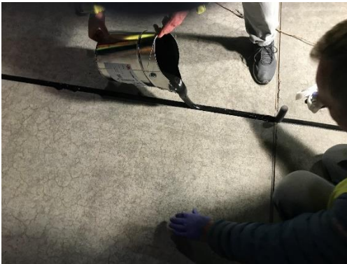
Picture 3: Application of Sikaflex-406 KC directly out of the pail
